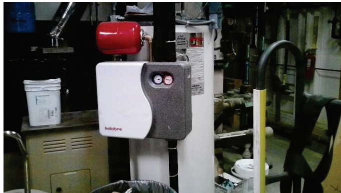
Heliodyne Heat Transfer Appliance and Solar Heat Exchange Tank
