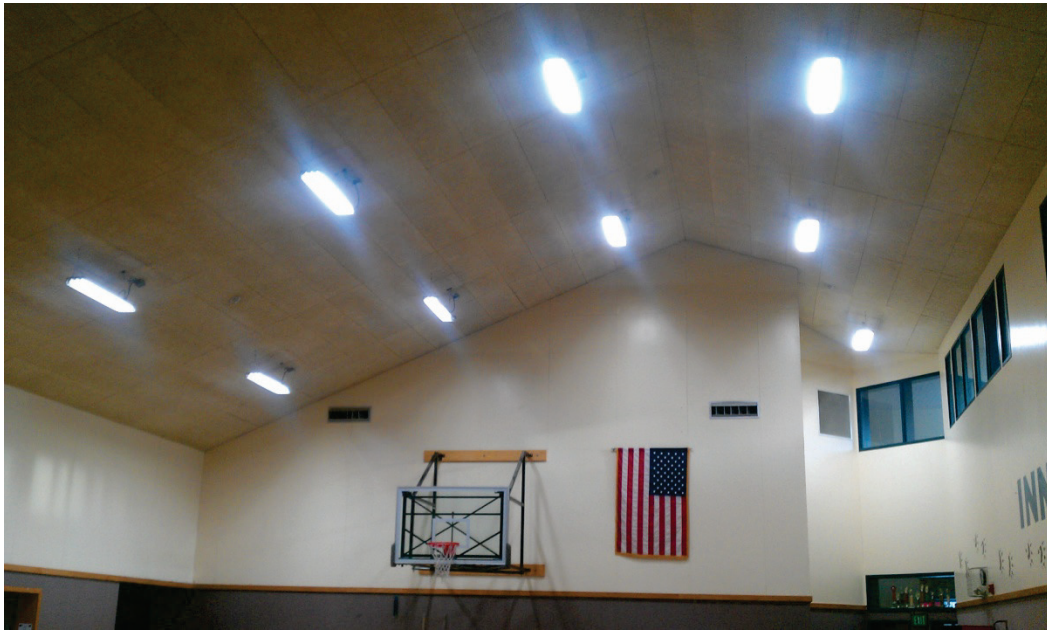
Completed T5 Installation
